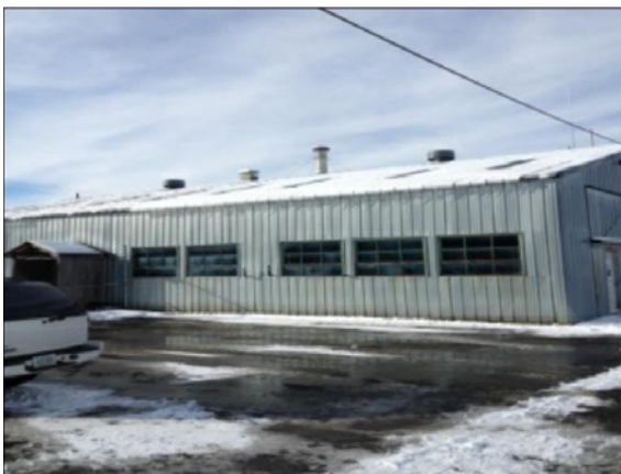
Maine DOT Storage Building
