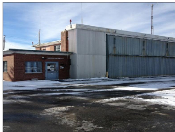
Civil Air Patrol Hangar
